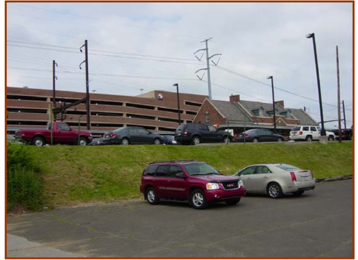
View of Adjacent Septa Parking Garage
